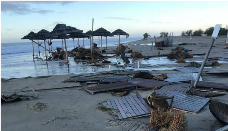
Figure 13: Damages to the beaches of Bibione caused by the storm surge event on the 1st of November 2021. Source: Il Gazzettino ( www.ilgazzettino.it )
